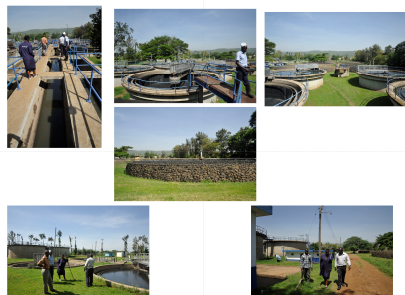
Sewage Treatment Plant Kisat: An old, but well operated trickling filter plant
